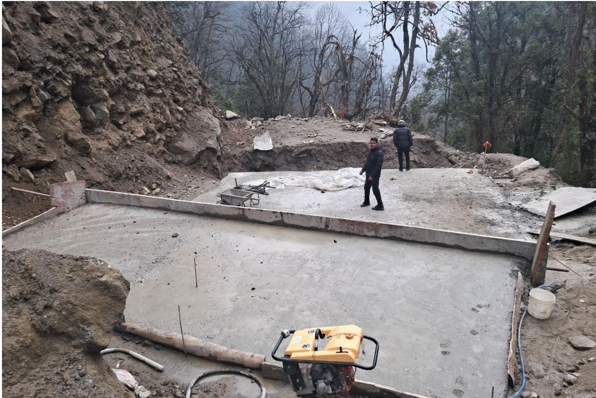
Figure 13: PCC work in Anchor Block 12 foundation
