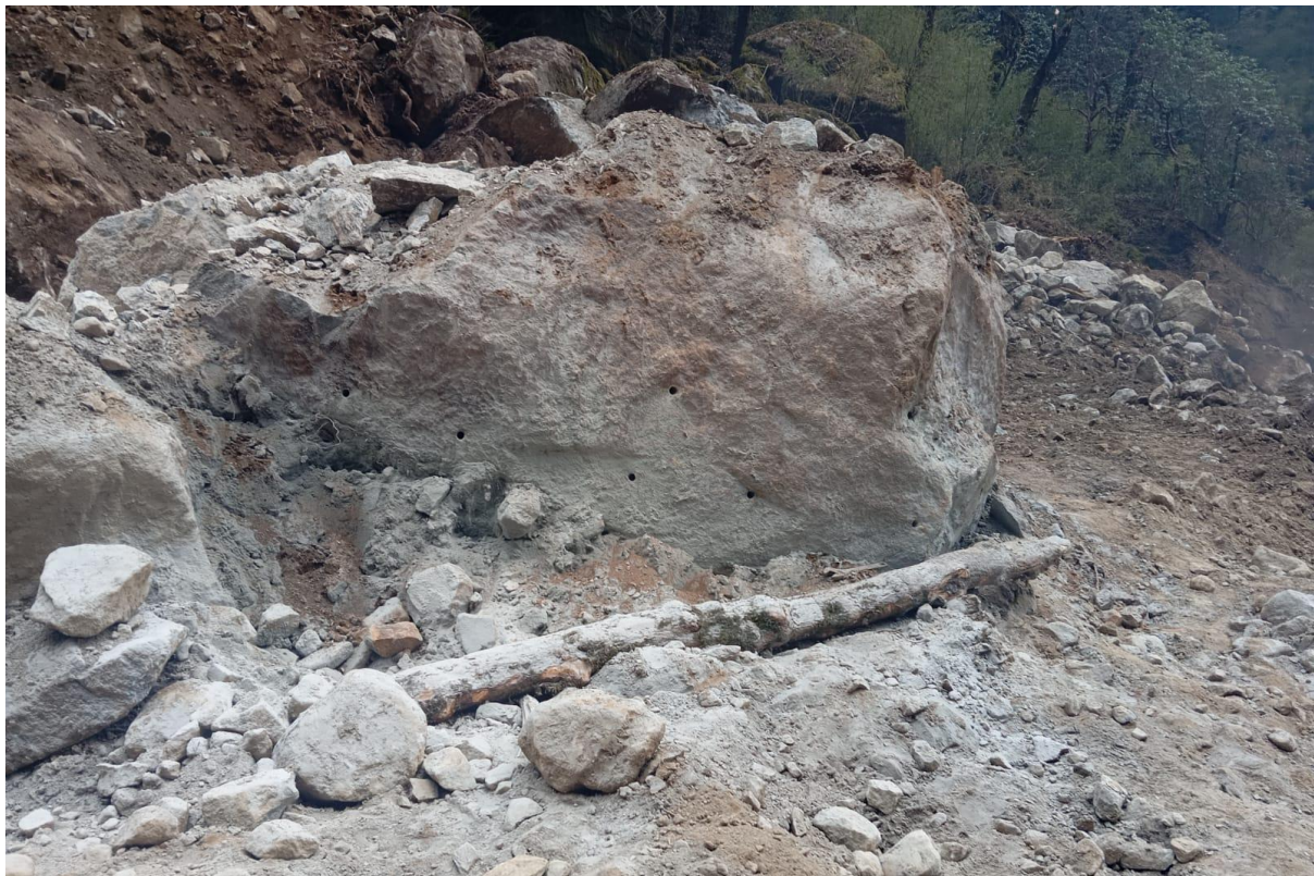
Figure 5: Drilling on boulder in Approach culvert area
