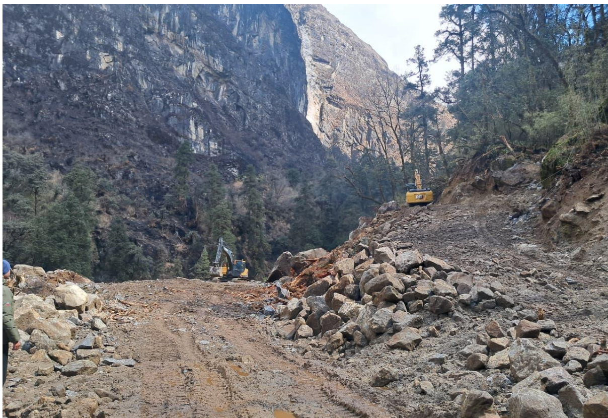
Figure 4: Earthwork excavation in Desander area
