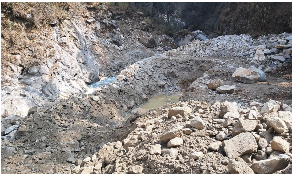
Figure 2: Headworks area (Undersluice)
