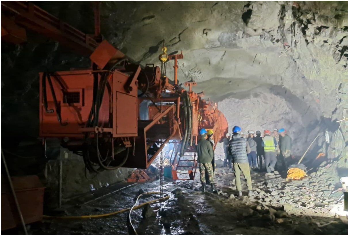
Figure 9: Raise climber installation
