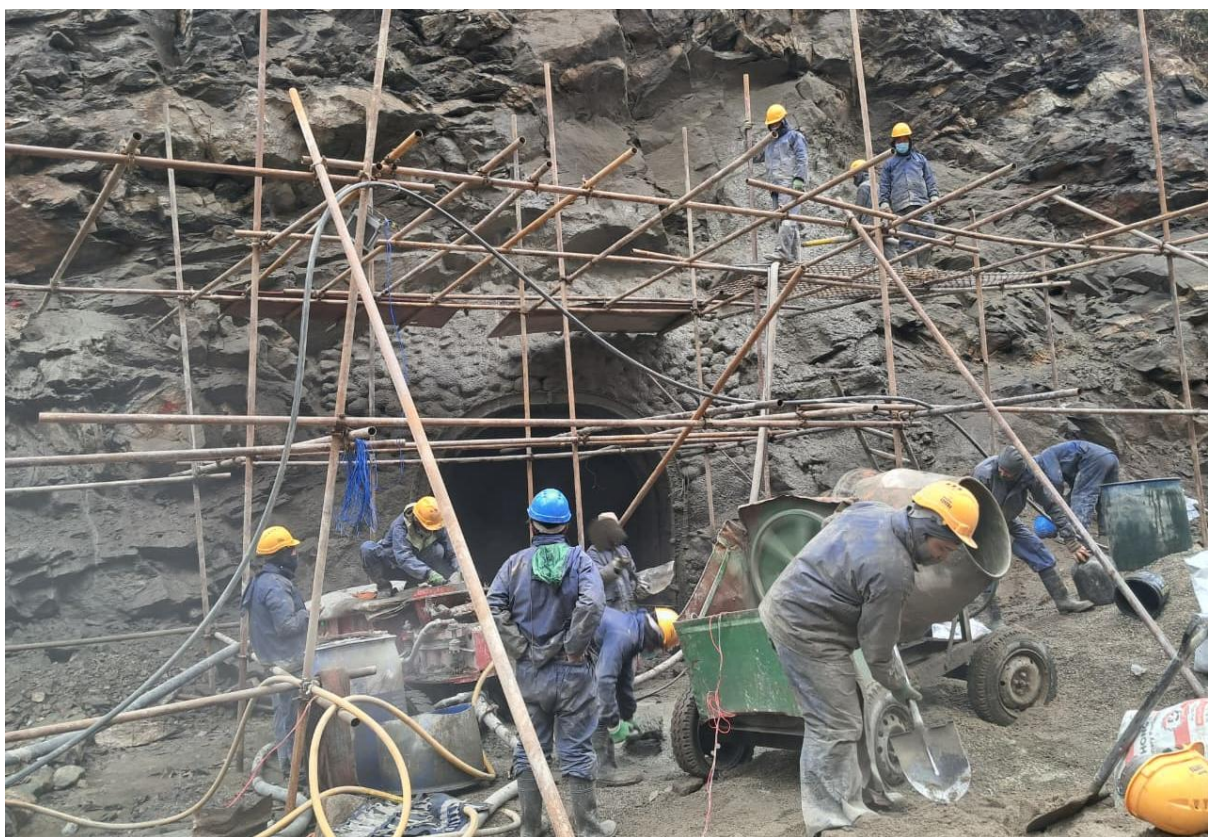
Figure 6: Shotcreting in HRT Inlet Portal
