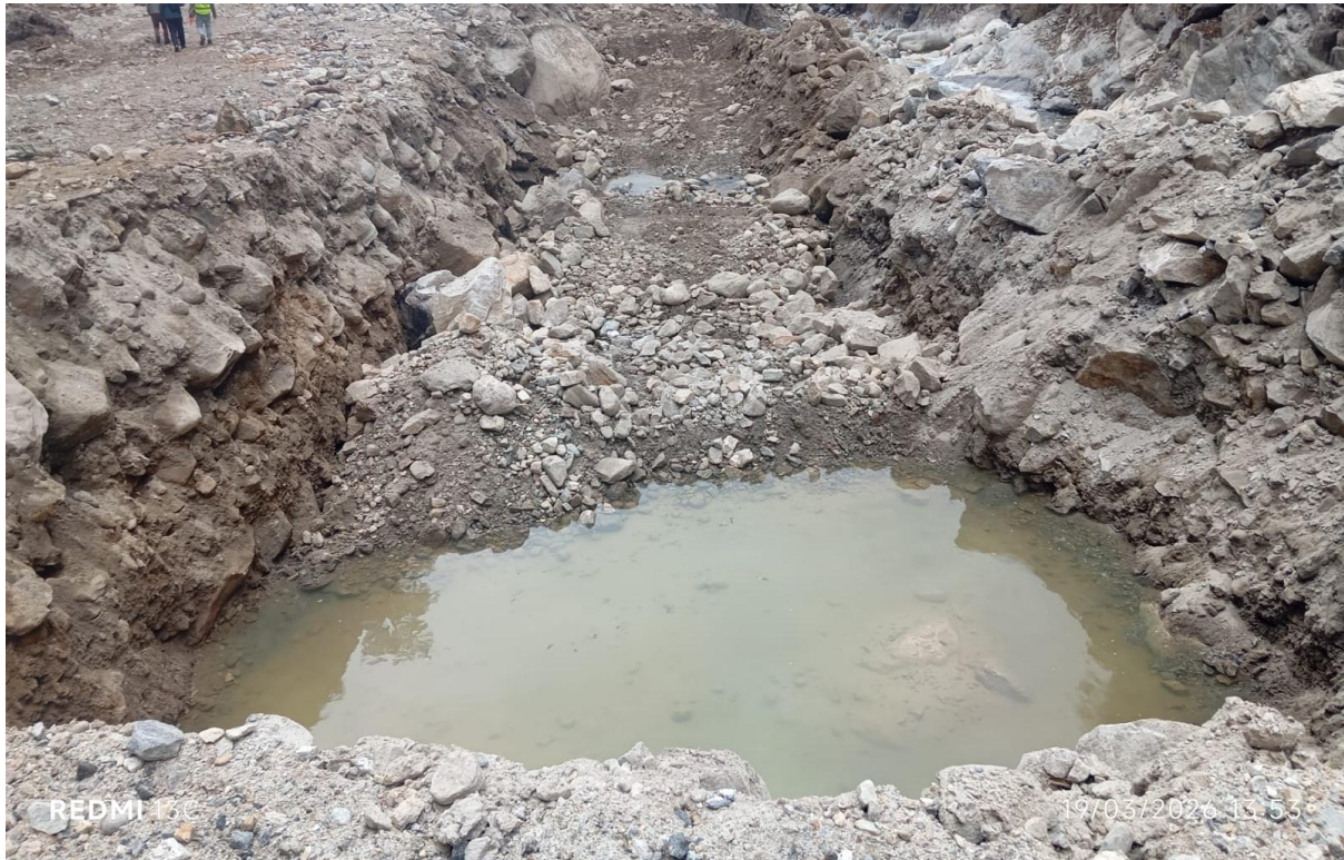
Figure 1: Undersluice excavation in Headworks Area
