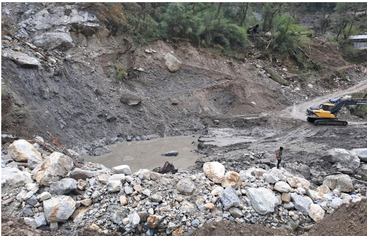
Figure 16: Excavation in Bridge left abutment foundation in new alignment
