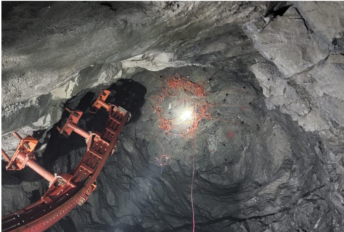
Figure 11: Preparation for blasting in Vertical Shaft
