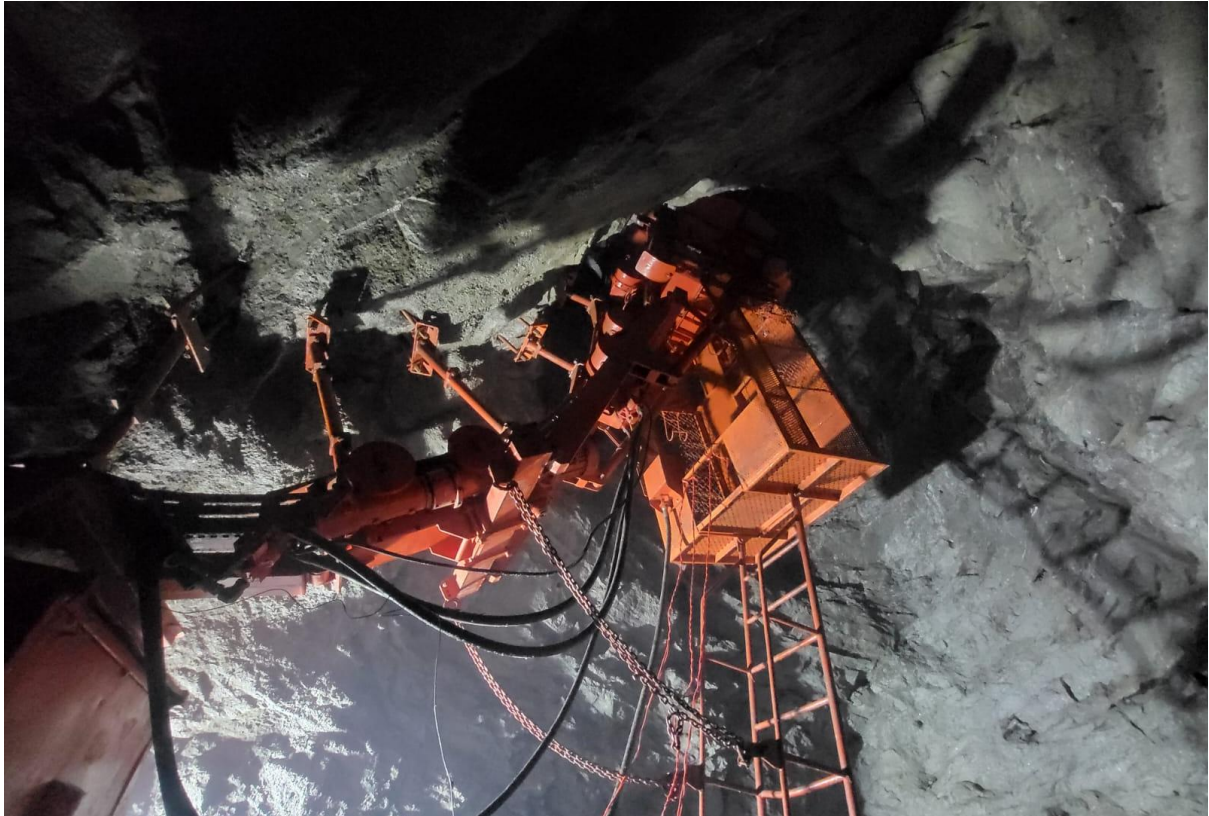
Figure 10: Drilling with Raise climber in Vertical shaft
