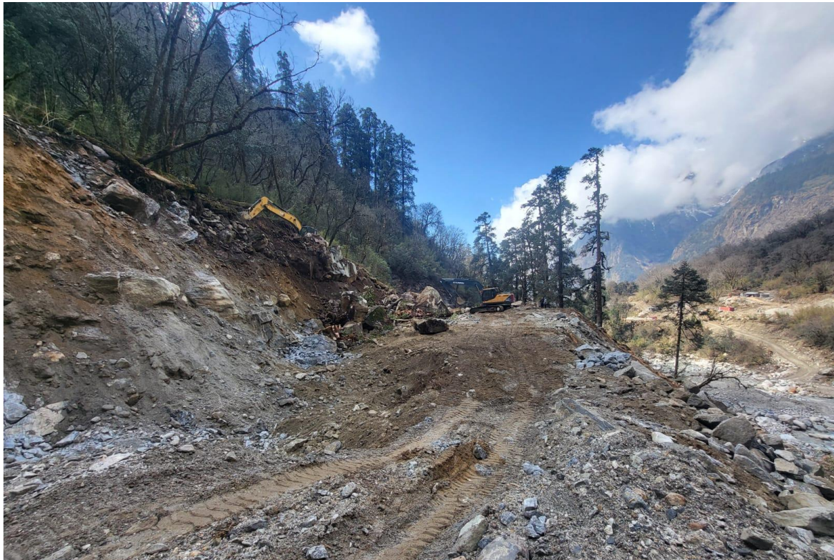
Figure 3: Earthwork excavation in Desander and Approach culvert area
