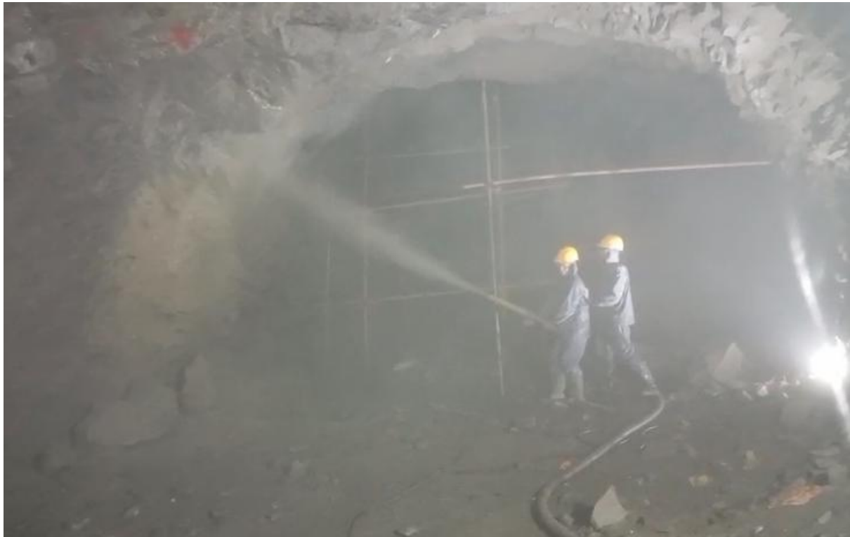
Figure 7: Shotcreting in widened part of Penstock Tunnel
