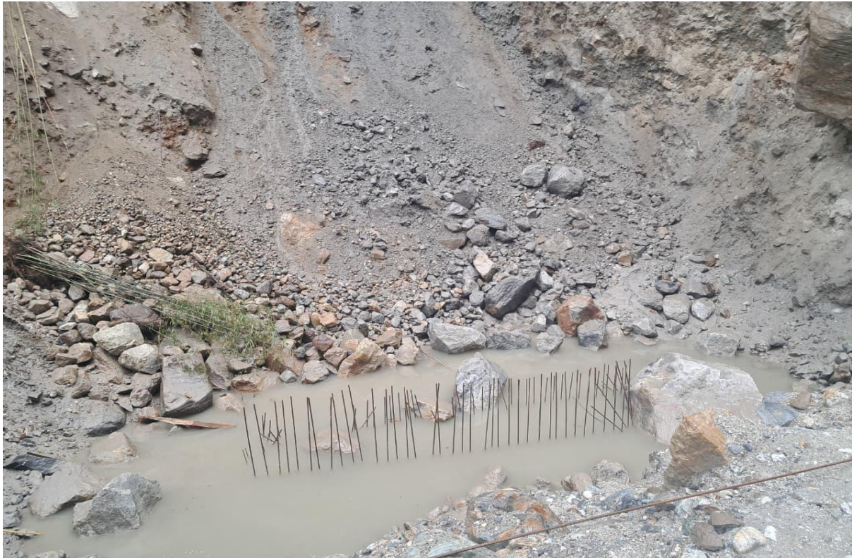
Figure 15: Surveying and base station development near Powerhouse
